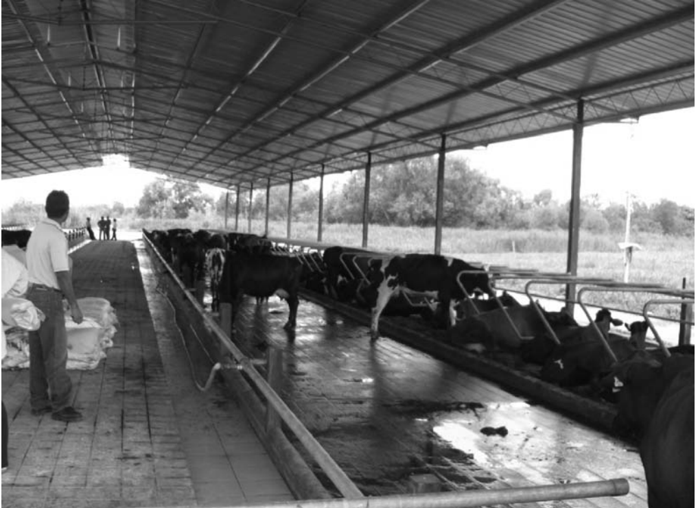
A well-planned free stall shed in Malaysia.
