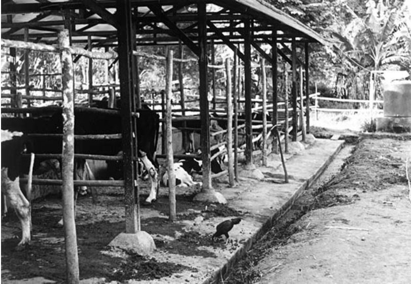
An all too common problem of slippery floors due to poor hygiene in a shed in Malaysia.
