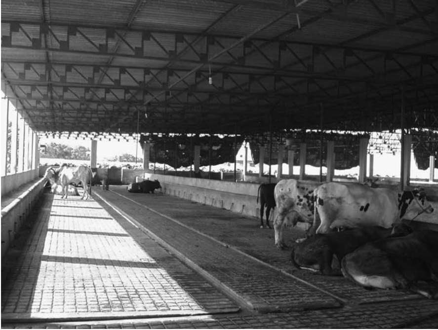
This is the shed for which the curtain was installed (Pakistan).
