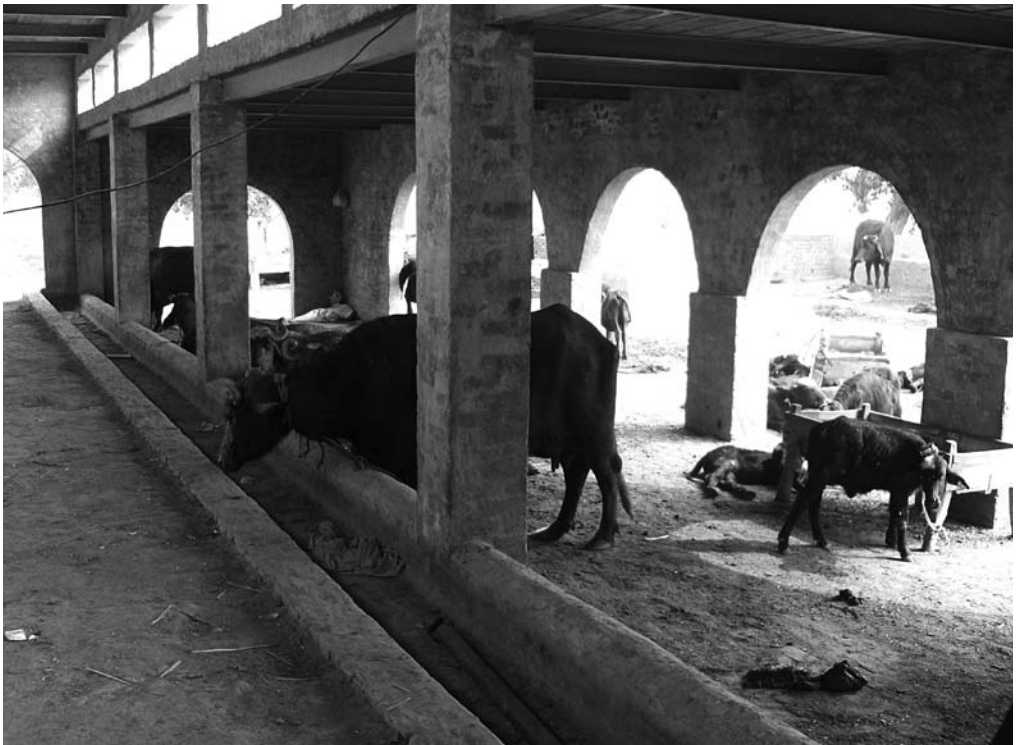
A well-designed shed under construction in Pakistan.
