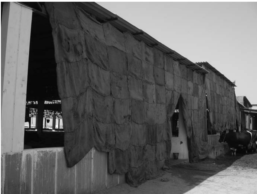
For some reason, this curtain was installed to reduce cold stress in coastal Pakistan.
