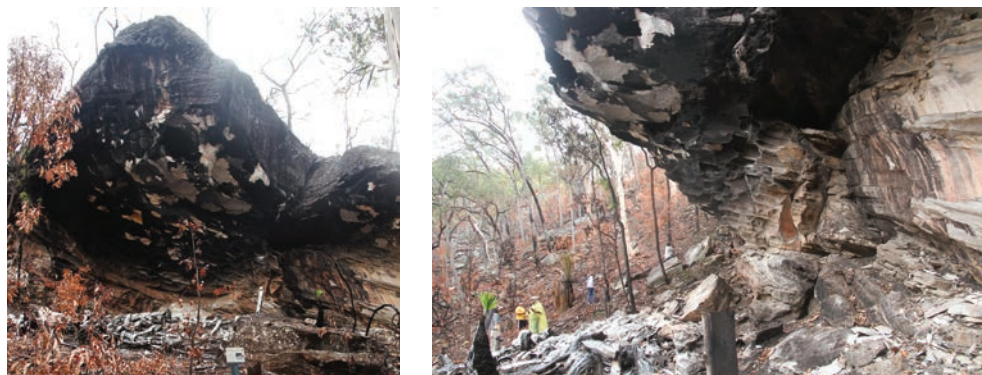
Fig. 3.1. Baloon Cave Carnarvon Gorge, Queensland after wildfire destroyed the recycled plastic viewing platform. The heat was so intense much of the rock shelter surface exfoliated and collapsed, destroying or severely damaging rock art. Black soot covered remaining parts of the shelter wall and ceiling. (Photos: Paul S. C. Taçon, Griffith University, Queensland)
