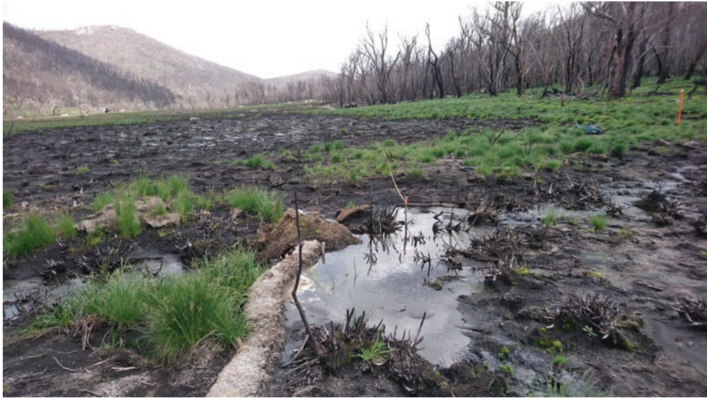
Fig. 8.3. Coir log damming the stream channel to slow and spread water throughout the peat soil, at Rotten Swamp in the Australian Capital Territory. (Photo: Nina McLean)
