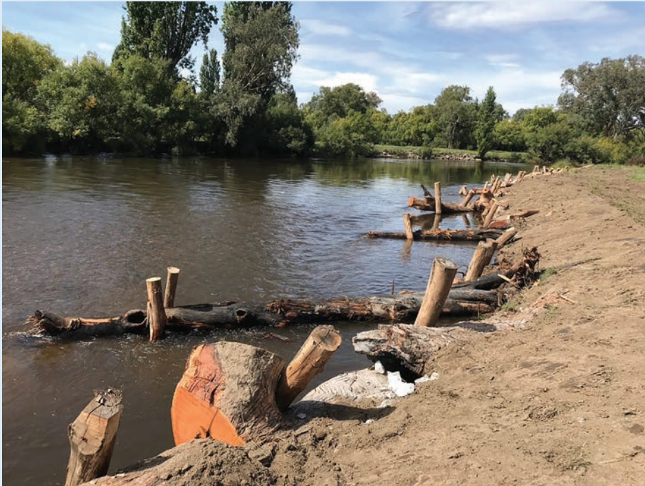
Fig. 25.2. Timber from wildfire-affected trees removed to maintain road safety used to control erosion and improve the habitat of the endangered trout cod. (Photo: David Thatcher)
