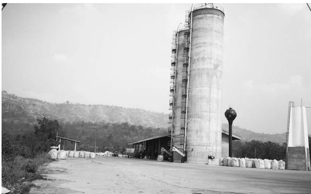
The Nong Yai feed centre managed by the Banbueng dairy cooperative in southern Thailand. This centre stores maize silage in tower and pit silos and prepares total mixed rations for delivery to cooperative members.
