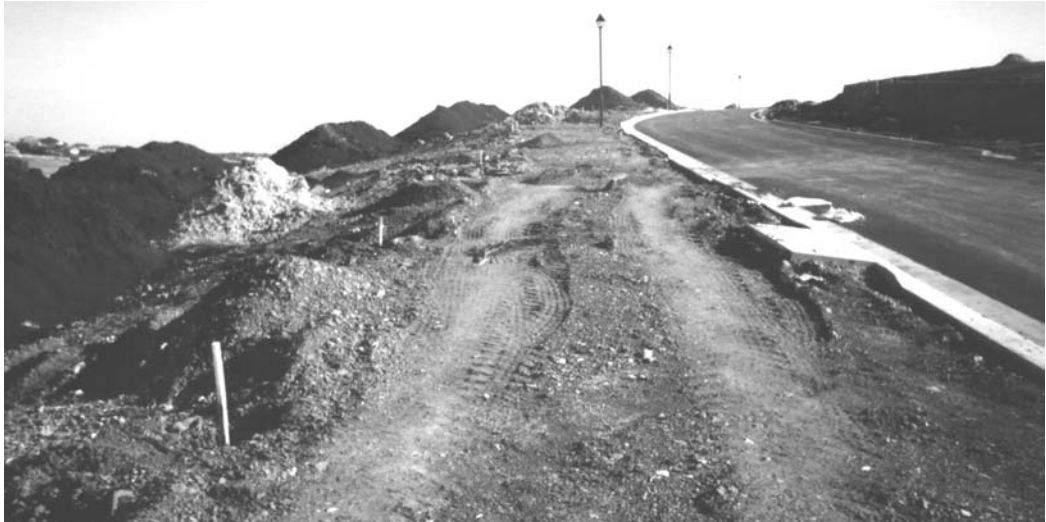
Figure 6.7 Land development results in significant vegetation removal and soil disturbance.
