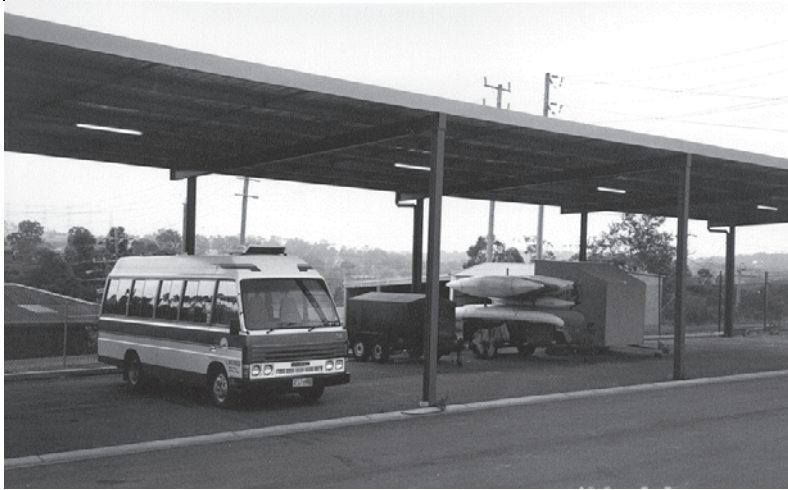
Figure 6.2 A temporary storage facility, undercover and with a spoon drain to redirect surface flow (City of Manningham).
