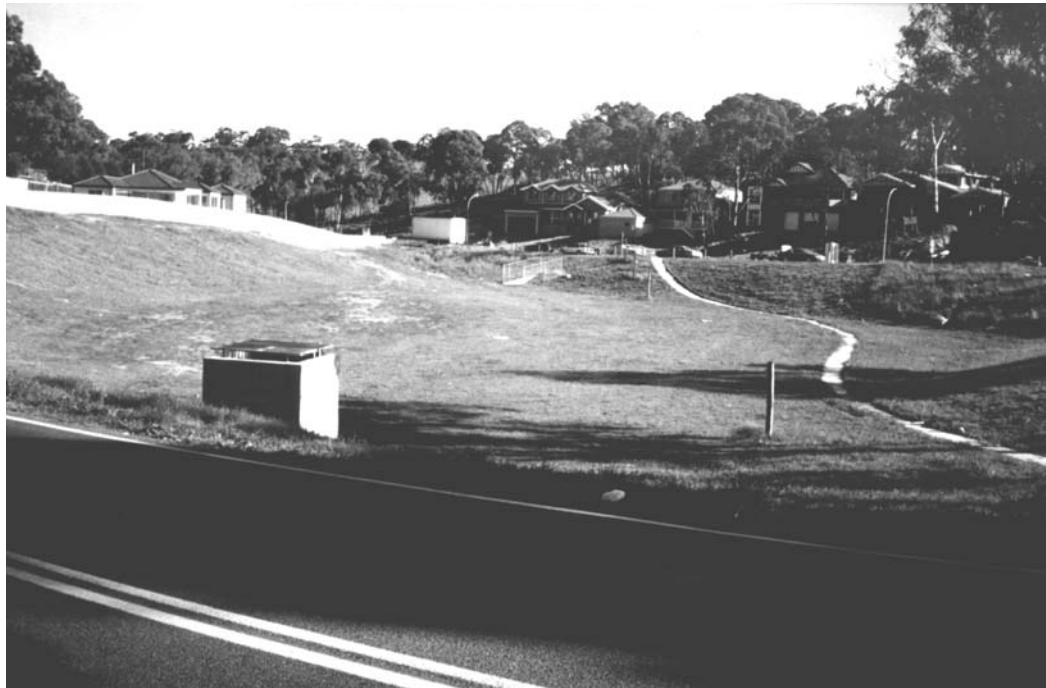
Figure 7.29 Extended detention basin.
