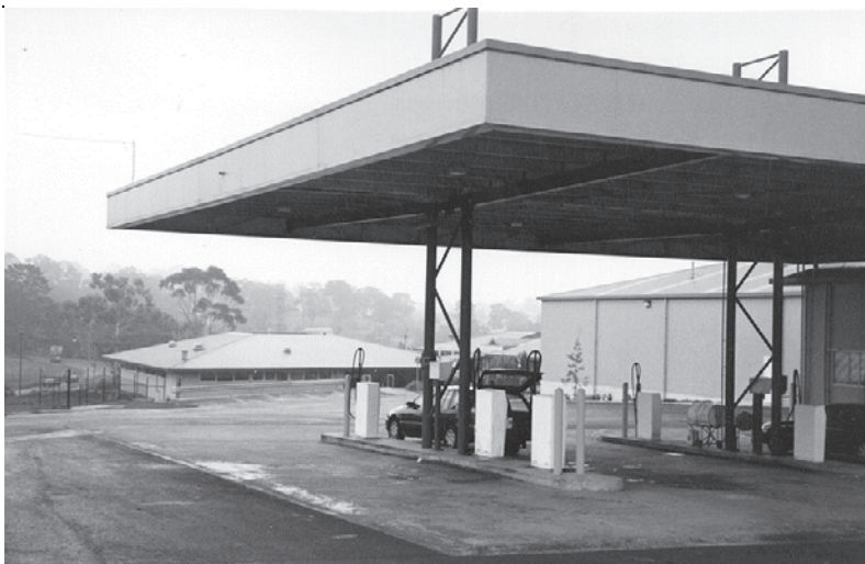
Figure 6.4 A fuelling area: paved, undercover area with a spoon drain to redirect surface run-off (City of Manningham).
