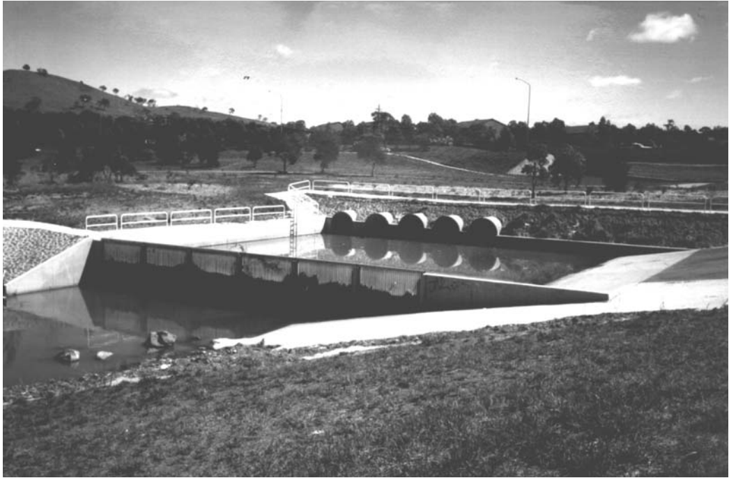
Figure 7.13 Gross pollutant trap, Tuggeranong Lake, Canberra.
