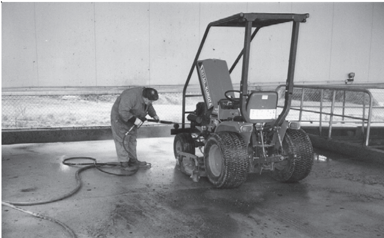
Figure 6.3 A designated wash-down area at the City of Manningham's works depot. A paved, undercover area draining to a sump (City of Manningham).
