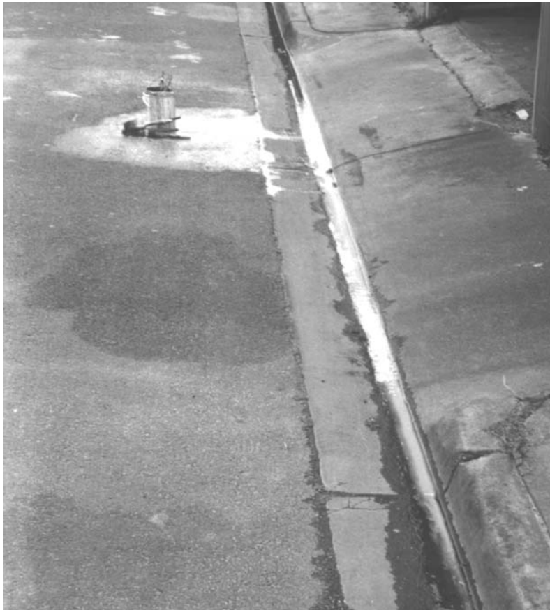
Figure 6.5 Many building maintenance practices can pollute stormwater.
