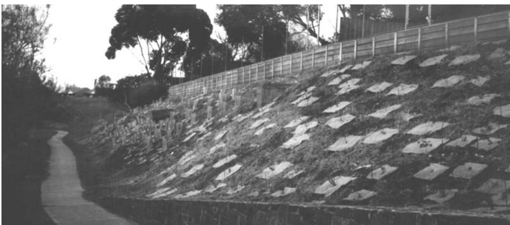
Figure 6.10 Stabilisation and revegetation protect soils from erosion.
