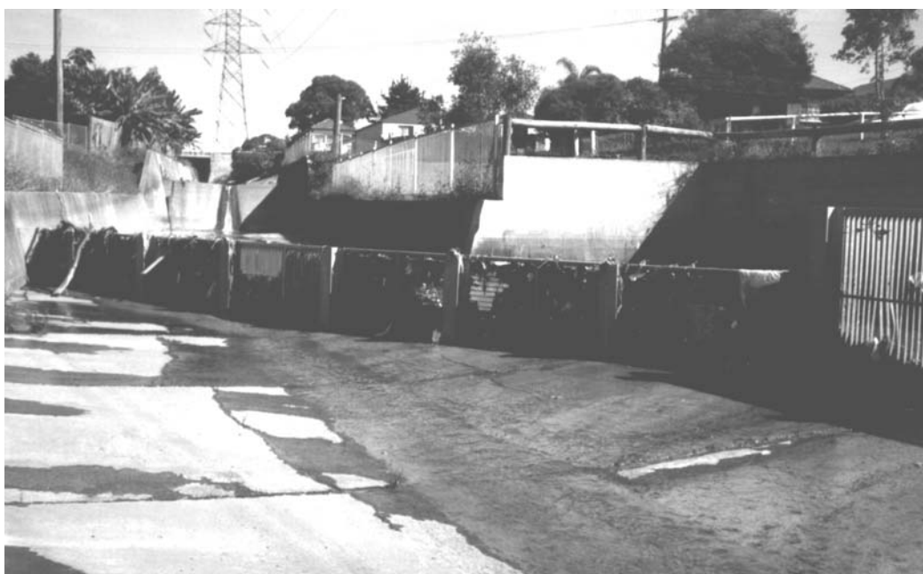
Figure 7.12 Trash rack (Cup and Saucer Creek, Sydney).
