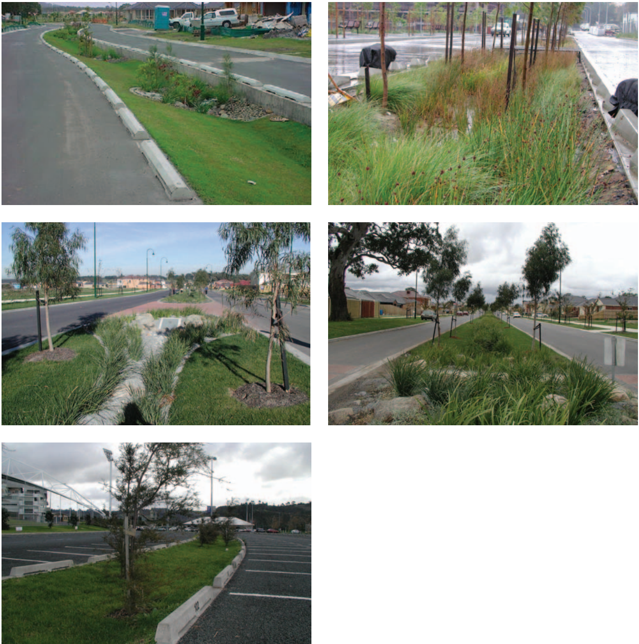
Figure 3.2 Bioretention swales are commonly located in median strips of roads and carparks
