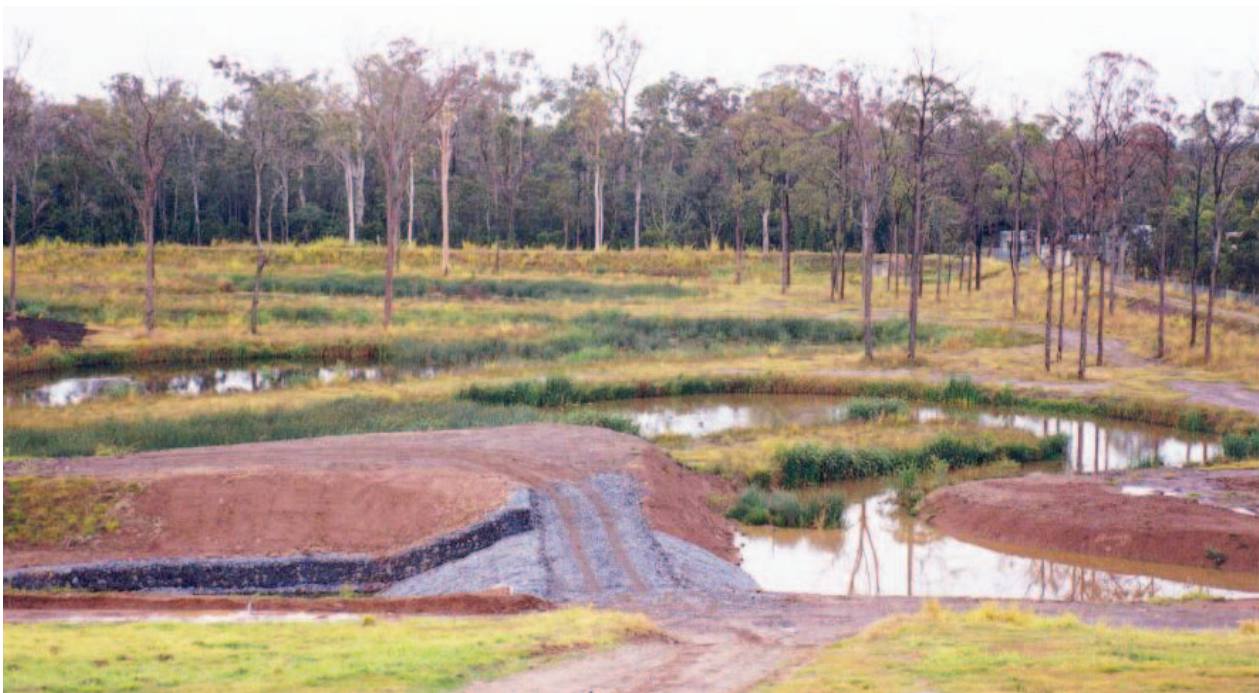
Figure 4.10 Overflow structure of a sedimentation basin.
