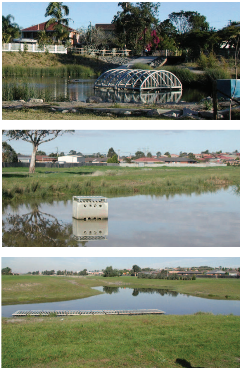
Figure 4.8 Debris protection for outlet pits.
