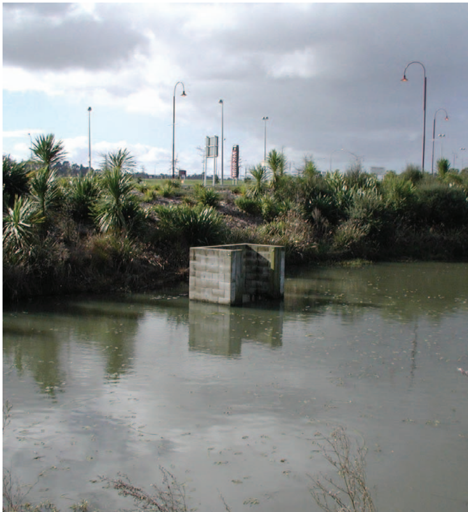
Figure 4.6 Sedimentation basin outlet structures: (a) a floating skimmer and (b) a narrow weir.
