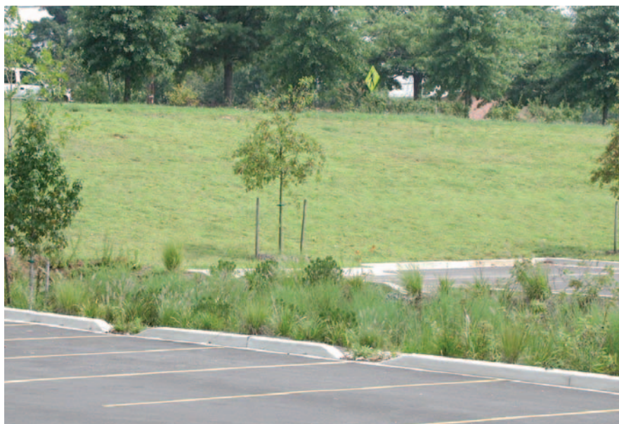
Figure 5.9 Kerbs with breaks to distribute inflows.
