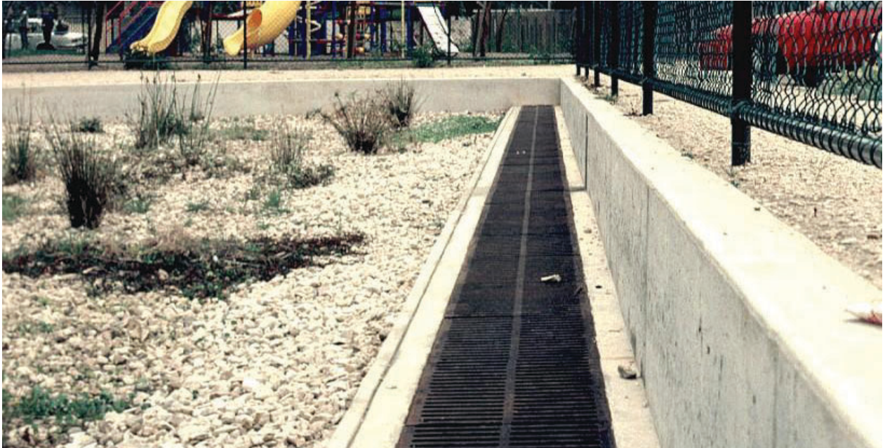
Infiltration system in Adelaide, showing the overflow trench
